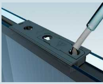
4. Fill the special openings of the module junction box in turn with sealant
