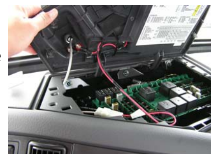
Tilting and Removal of Top
